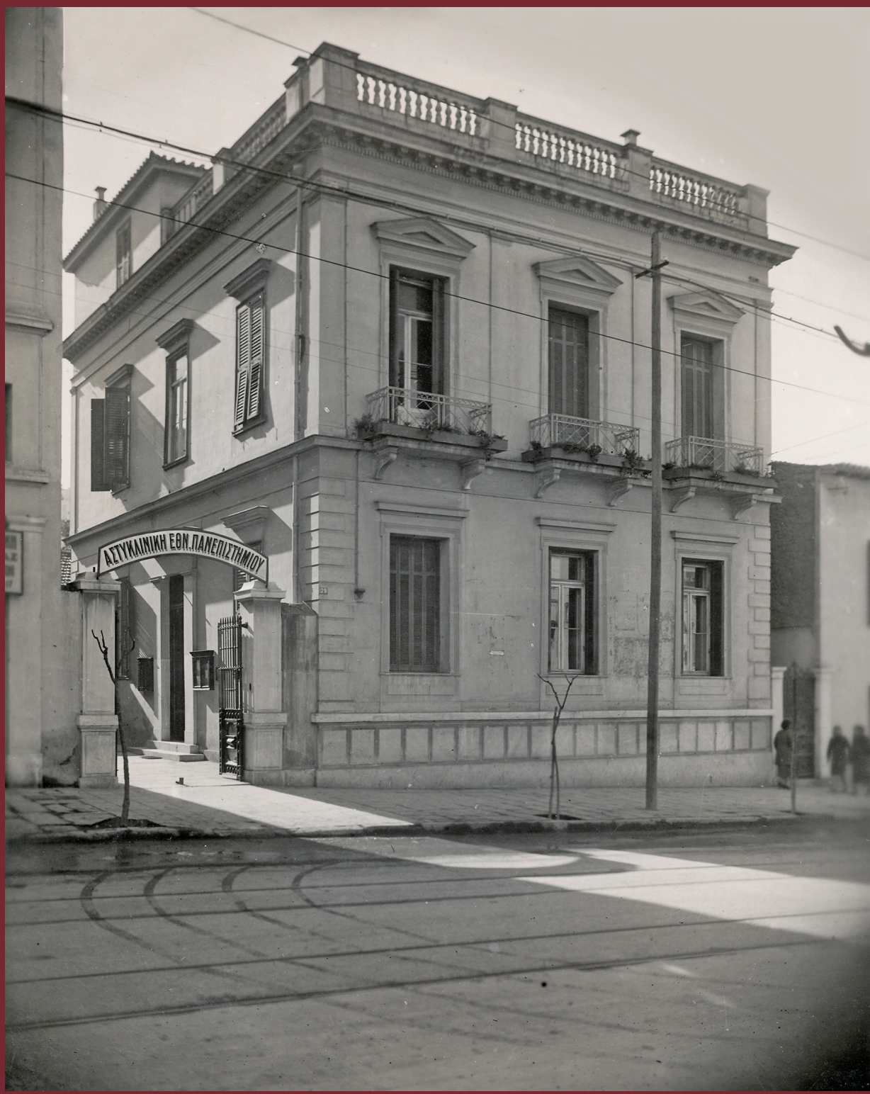
The building of the Clinic of the National University (Astikliniki) on Pireos Street, 1930s.
